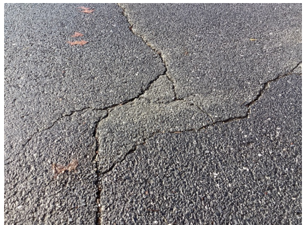
2004 pavement cracks
