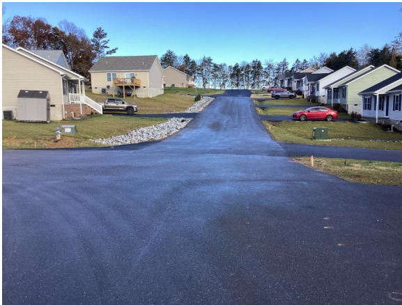
2019 asphalt pavement street overview
