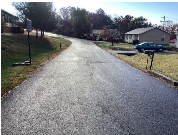
2004 asphalt pavement street overview
