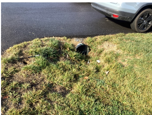
Metal culverts overview
