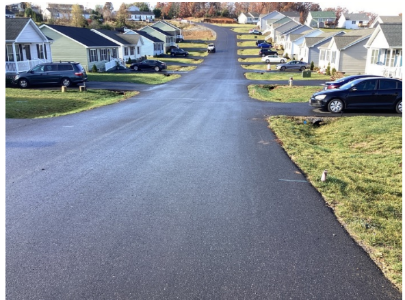
2019 asphalt pavement street overview
