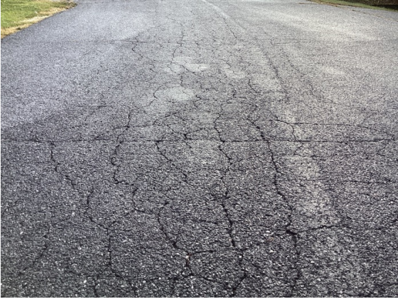
2004 alligator cracking
